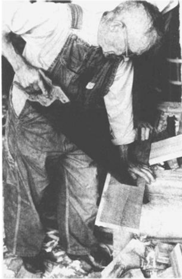
ILLUSTRATION 28 Cut off the board piece with a handsaw.
