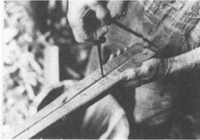
ILLUSTRATION 10 Alex uses a compass to mark his gauge for different-sized churn heads.
