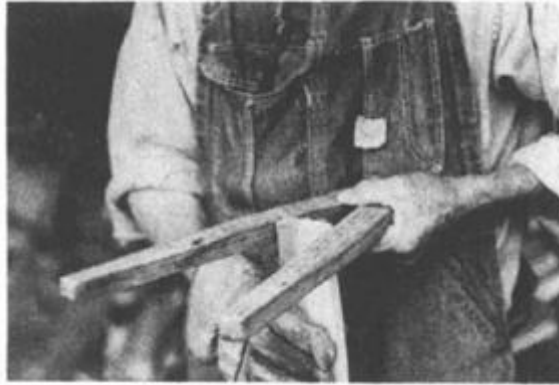
ILLUSTRATION 13 Alex checks his stave angle on the gauge. The correct angle should be maintained as closely as possible for the full length of the stave. However, the angle does not have to be perfect. The wood, being pliable, seats itself. The last stave to be fitted ( Step 5, ILLUSTRATION 18 ) has to be driven into place. This closes most of the cracks which may result from slight errors in the angles of the other staves.
