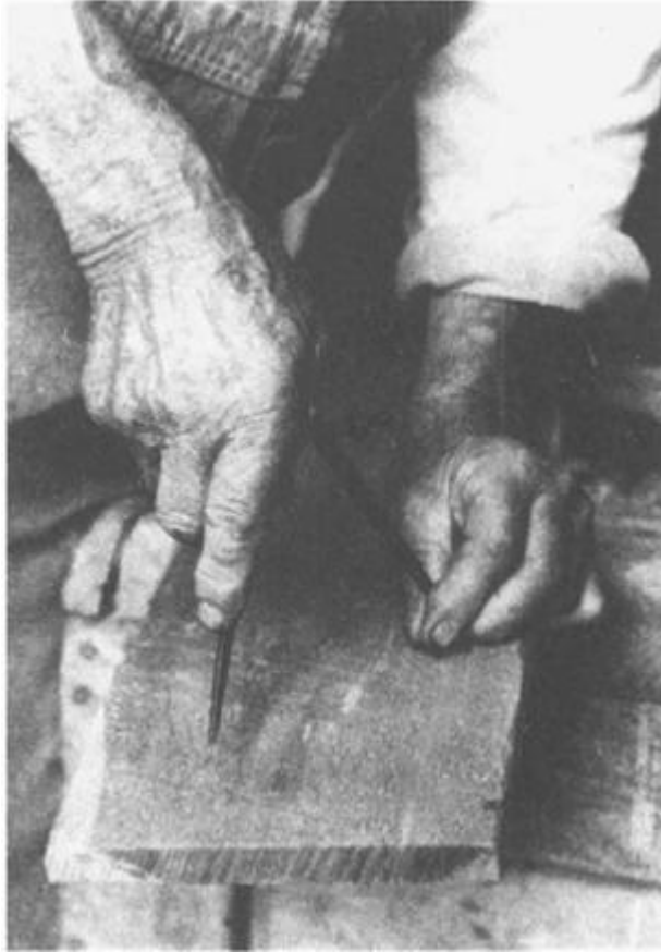
ILLUSTRATION 27 Step 10: Use cedar board(s) for the head (the bottom of the churn). Use any size board and as many pieces of board as needed to make the proper size circle. Use a compass to mark the proper size.
