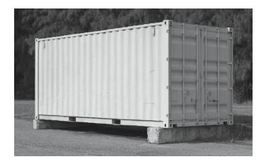
The first problem is that containers are essentially a hardened skeletal frame with sheet metal skirting. They are made to stack under extreme loads, but the sides rarely touch anything. Because of this and the need to keep shipping weights at a minimum, the sides are hardly much more than hard curtains. In fact, a simple bump by truck or tractor will dent or even tear the siding.
