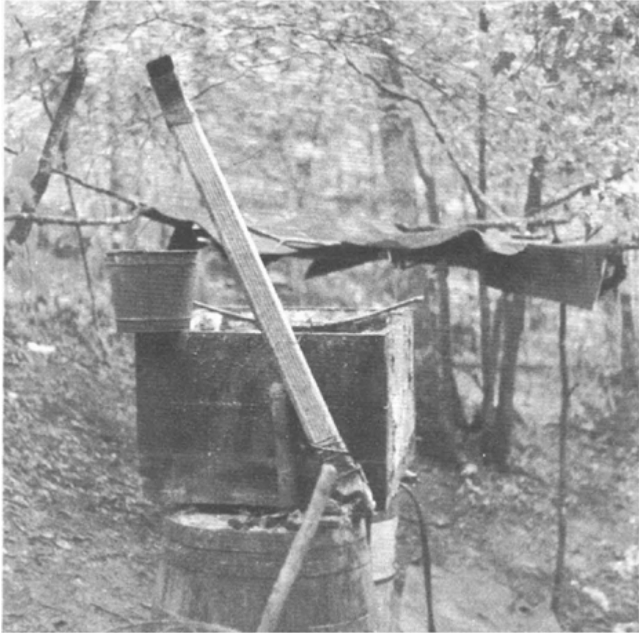
ILLUSTRATION 15 The thump barrel and heater box. The drain pipe, when lowered, carries warm, fresh beer from the heater box to the cooker, the top of which is visible in the foreground.
