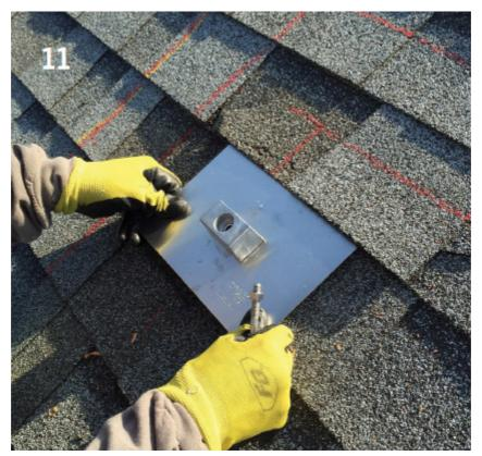
12. In the photo, we can see the installer has inserted the steel flashing into position between the shingles.
