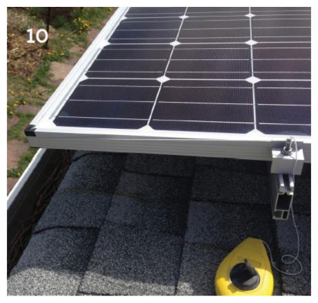
11. Here, in the photo, we can see the installer has tightened the alignment string marker the entire length of the bottom row, which will facilitate aligning all the panels in the bottom row to be parallel with the edge of the roof and parallel with each other.
