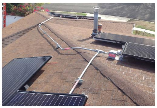
The conduit wiring from the micro-inverters across the roof and down to the electrical control equipment.
