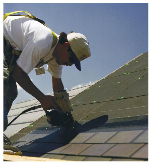
The installer is securing this thin film array onto a very steep roof flush with the roof surface.
