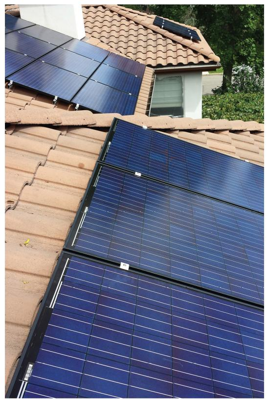
Two poly arrays on two different slopes of the same roof.
