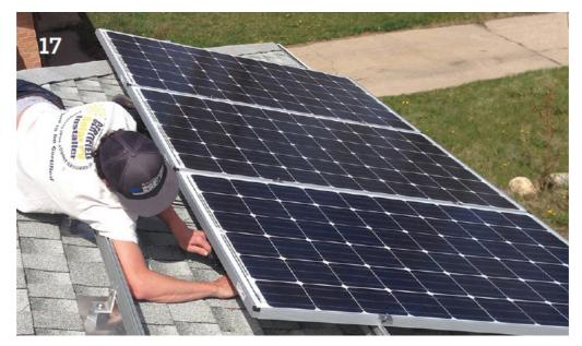
18. As shown here, it can be a bit of a tight fit to make the final connection between the leads of adjacent PV modules but the mounting support frames are engineered to allow a normal size person or worker to reach under the modules and complete the task of wiring the system.
