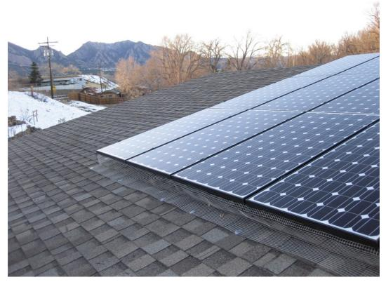
A small array of mono panels mounted flush to the surface of a wooden shingle roof. Wood roof shingles are normally made of cedar that has a natural attractive finish and they have a long useful life to match the expected useful life of PV panels.
