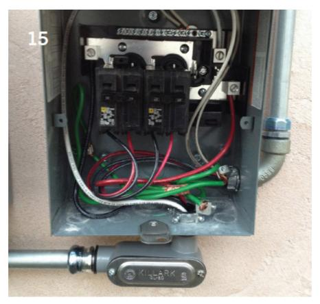
16. This photo shows the AC combiner panel all wired up with its face plate attached.
