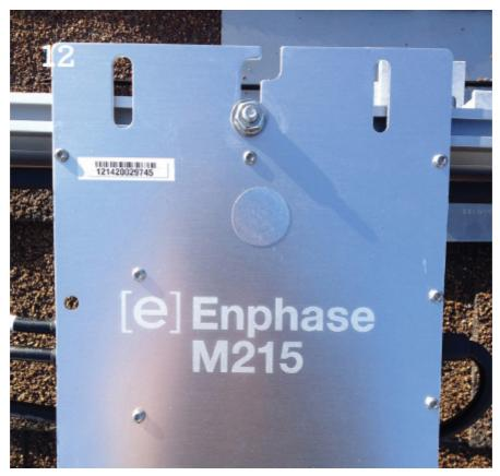
13. The photo shows a small micro-inverter with its 2 leads ready for connection. When micro-inverters are incorporated into each PV panels, you can find them installed on the backside of each module along the upper edge right-hand corner and they are not visible after installation from the side or from above.
