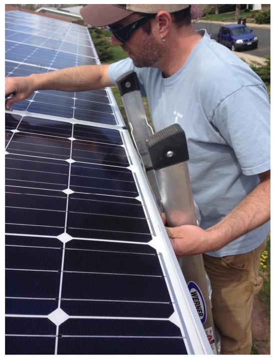
A DIY installer inspecting his mono panels up on an aluminum ladder. This kind of ladder is not recommended for use when wiring the PV rooftop system as it can conduct electric current. I always insist that DIY PV system installers use only wooden ladders.
