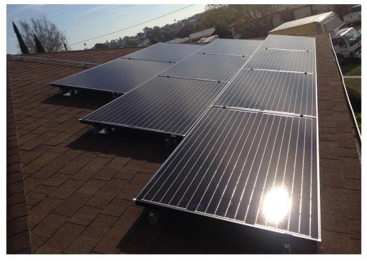
Nine poly PV modules mounted after having the micro-inverters connected from the support rails and then to the modules.
