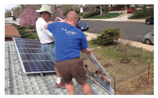
2. In the photo, the DIY installer's assistants are helping the delivery truck and crane to unload the solar PV modules and rails at the job site. These workers should be wearing construction hard hats and for safety should avoid standing directly under the load.
