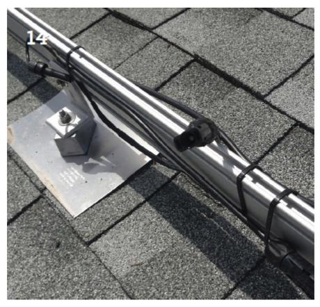
15. This close-up photo shows a male and female connection that have been attached to one another and this line is labeled as part of "string 1" that includes the 13 modules of the bottom row shown in the photos above.
