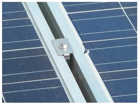
A close-up shot of the mid-bracket securing two poly panels to the support railing below (not visible here).
