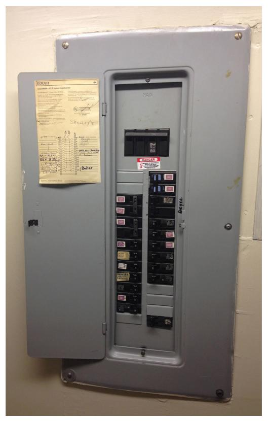
The main electrical panel for the house. In this case, there is a grid-connection via a back-fed breaker in the panel. While this does serve as a disconnecting means for the panel, utilities generally require a separate, accessible, dedicated AC disconnect switch such as those illustrated earlier in this chapter under the heading "DC and AC Disconnect Switches."
