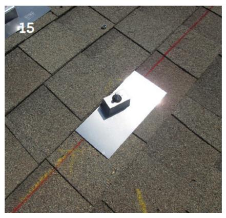
16. In the photo, the installer has just prepared the steel support bracket for drilling through the flashing to the roof
