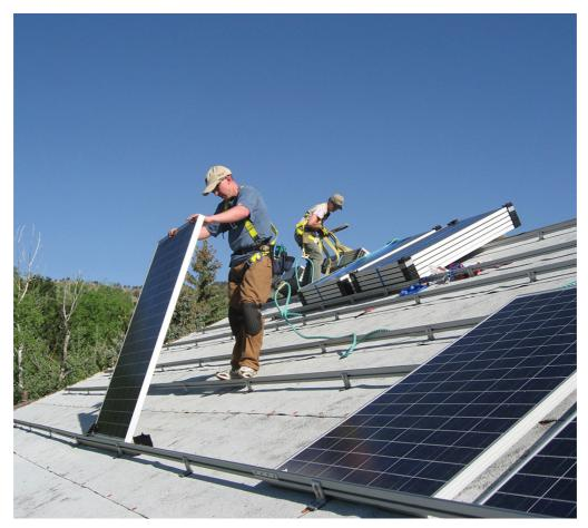
Two DIY installers start to install a large number of poly panels on a low-tilt roof of white asphalt tiles. You will notice that the aluminum rails of the solar system support structure have already been completed without any additional tilt.
