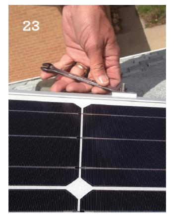
Also, in the photo, we can see that this PV installation is using monocrystalline silicon PV modules as opposed to polycrystalline silicon modules. The differences in appearance and performance and the various pros and cons of these two types of modules are discussed and illustrated in Chapter 1.
