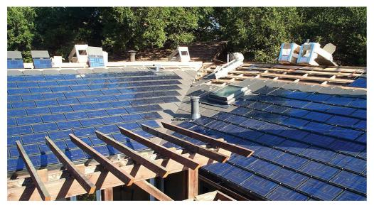
In this photo, we can see the solar PV system is being installed at the same time as the installation of a new roof.
