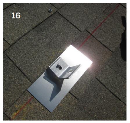
17. In this photo, we can see the DIY installer is midway through installing one of the steel support brackets.Vertical supports will then be attached to a horizontal support railing. In this way, all the vertical supports will connect the horizontal railing to all the support brackets as illustrated in the photos below.
