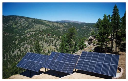
Three arrays of 12 poly modules, each that are ground-mounted on three terraces in steep terrain. When your rooftop space is insufficient for your solar power requirements, this type of ground-mounted supplementary PV installation may be a good solution if the extra space is available somewhere behind your house.
