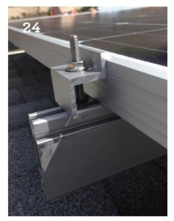
25. In the photo, we can see that the DIYer has installed one of 2 mid-clamps, getting ready to install the next panel parallel to the panel already installed.
