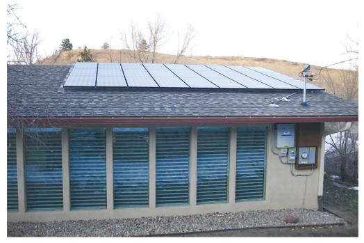
A low-level rancher with an array of 11 panels mounted flush to the roof surface.
