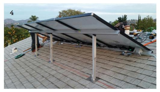
The small array above of 4 modules may be additional to modules installed on the other side of the roof to increase total system production, or, on the other hand, the main array might be mounted on this side to avoid a shading problem on the other side.
