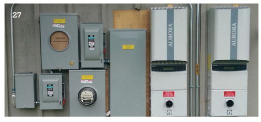
28. The photo shows the setup of the equipment area of a third, relatively simple PV solar system. Most of the same equipment items in the previous two systems are repeated here with only a few exceptions, but in this installation the current will flow from right to left.
