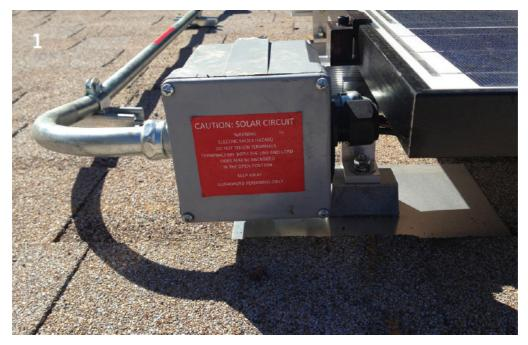
2. The photo is taken from the other side of the junction box and it shows how the DIY installer can use the conduit and a 90-degree conduit fitting to penetrate the roof. Notice the use of silicon to weatherproof the holes. The alternative is to feed the homeruns directly through a weather-head.
