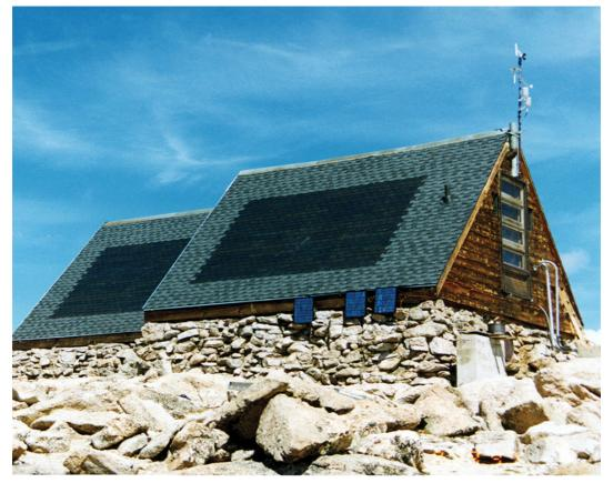
An attractive example of BIPV with the PV solar system installed on this very steep, two-roof house in Colorado where there is often big snowfalls in winter.
