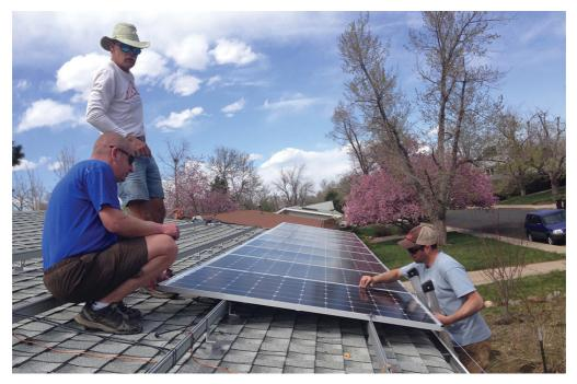
Here, we can see a do-it-yourself crew of three installing mono panels on the aluminum rails of an array that aligns very close to the edge of the roof just above the eaves trough.
