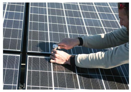
Here we see the installer tightening a mid-bracket between two poly panels and securing them to the railings of the support framework.
