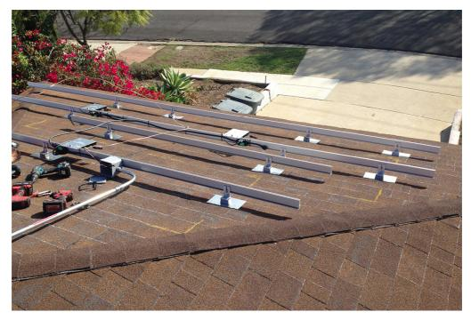
A side view of the same three rows of support rails mounted on the roof with microinverters already attached.
