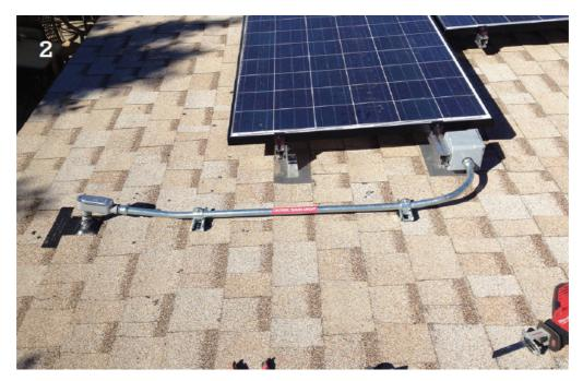
3. The photo shows how the DIY-install crew makes a 90degree bend in the conduit tubing without the need to connect or disconnect interior wires. This part of the conduit is held in place by a steel flashing, clamp, and lag bolt.
