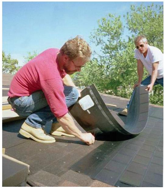
Two DIY installers holding a long, amorphous silicon thin-film panel that can easily adapt to a curved substrate or surface.
