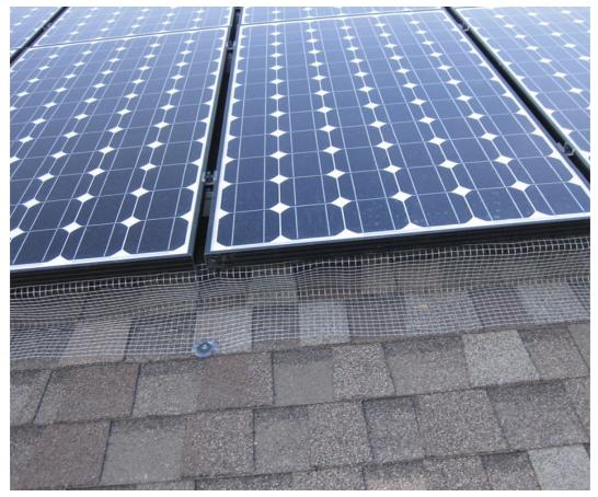
A compact array of six mono panels installed flush with the roof surface—a very typical mounting.
