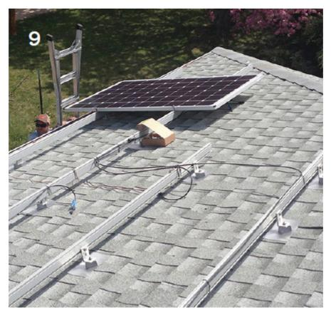
10. In the photo, we can see that the install crew is getting ready to attach a "tension string marker" for the purpose of aligning the bottom row of modules. This process is continued in the next photo.
