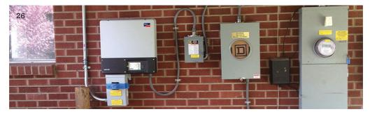
27. The photo shows a second system that is slightly larger than the system shown in the previous photo because it has two central inverters instead of one.
