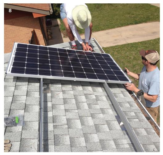
9. In the photo, the DIY installer has selected the approximate position for installing the end module at the opposite end of the bottom row of the array.
