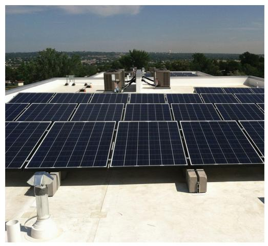
Numerous solar arrays with over 50 panels mounted on a flat condo rooftop with a tilt of about 20 degrees indicating that this installation is in a location with a latitude of about 20 degrees.
