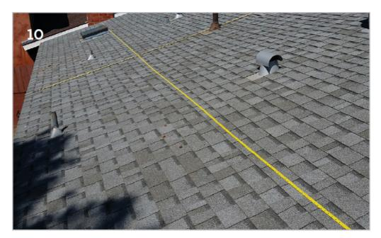
11. In the photo to the right, we see the DIY installer is taking and recording careful measurements from the edge of the roof to all the built-in roof obstructions. These measurements will enable the installer to prepare a drawing with an optimal and accurate layout for the panel array.
