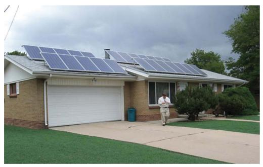
Four arrays of five poly modules, each installed with two arrays on the main house and two equal-size arrays on the garage. We can see that the roof has a tilt of about 30 degrees and the arrays are mounted with an additional tilt of about 15 degrees for a total tilt of about 45 degrees, indicating that this house is likely located near
