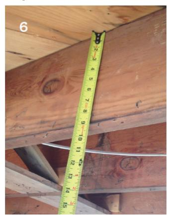
7. In this photo, the installer is measuring the spacing between structural members. In this case it is a standard 16 inches between centers. With these two measurements we can easily find the load bearing capacity of this roof per square foot. To determine the load limits for specified open areas, we also need the length of the open beams between vertical supports. Standard load bearing tables will give us the answers. The lumber supply depot supplies tables with this load bearing information.
