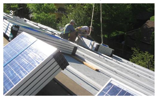
This is a fairly large installation but for smaller systems, the installer and his crew will often manually raise the PV modules up to the roof one by one using a ladder.
