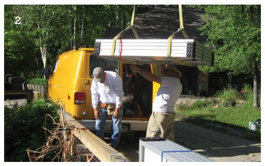
3. In the photo, we see the DIY installer and his crew guiding the crane driver and unloading the PV module packages onto the roof from the truck below. Notice that the horizontal support railings have already been installed and provide a bracing to prevent the module packages from sliding down or falling to the ground. A precautionary note: Be careful not to unload your module bundles in an unsafe position or on a dangerous slope of the roof where they might slide down and get damaged.
