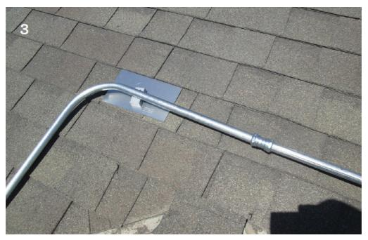
4. In the photo, we can see the DIY-install crew is attaching the conduit to a flashing with a lag bolt, spacer, and clamp.
