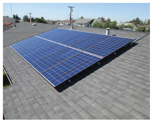
A very typical PV solar rooftop installation of  $(2 \text{ rows} \times 6 \text{ panels}) = 12 \text{ poly panels}$  that would qualify for optimal government incentives in most states of the United States.
