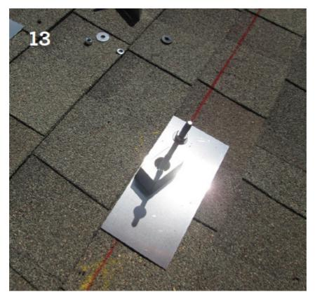
14. In the photo, our DIY installer is in the process of installing a lag screw into the roof support beam below the shingle. The lag screw will provide strength to the support framework rails that will be attached to one or several solar modules. (See additional photos below.)
