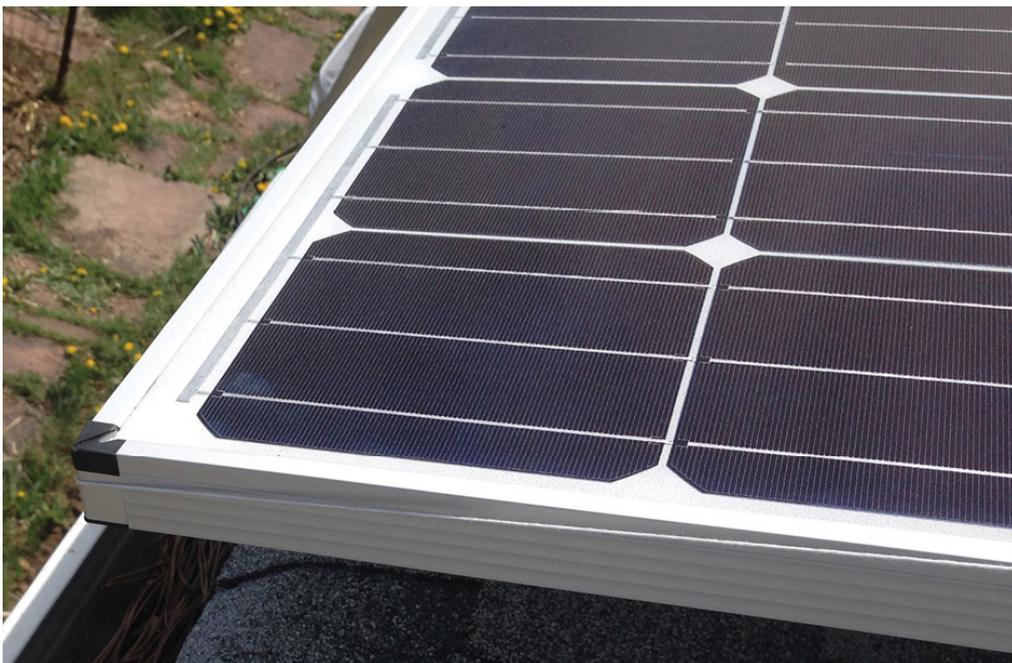
*A close-up shot of the corner of a mono panel at the end of an array.*
