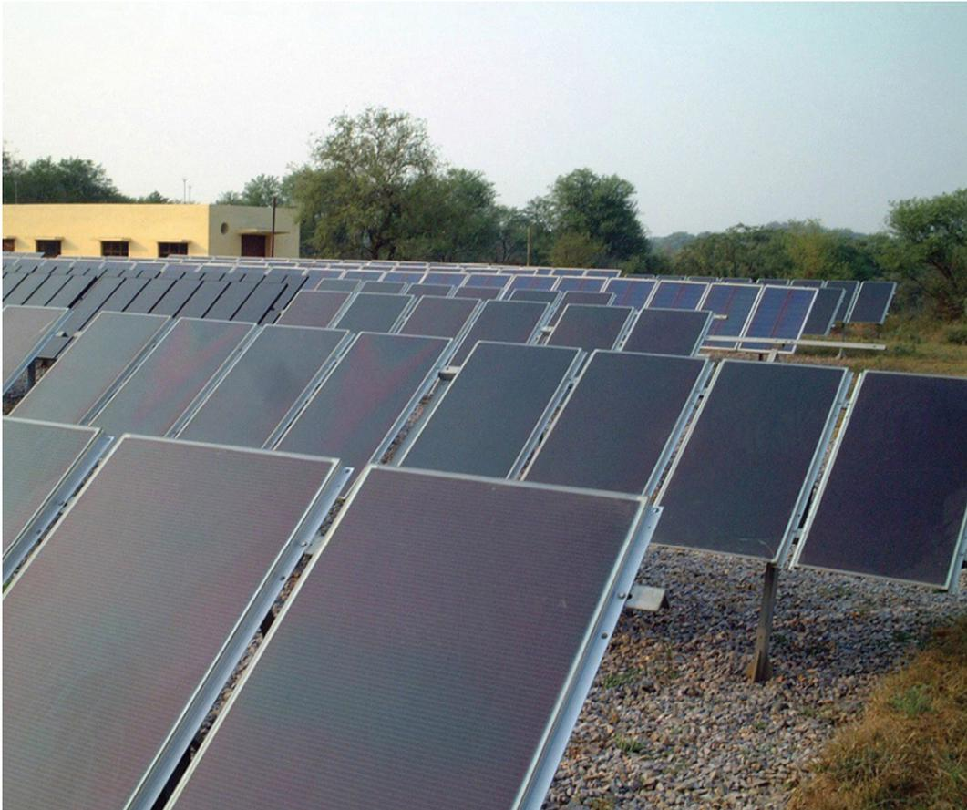
*A fairly common ground-mounted thin-film PV solar farm.*
