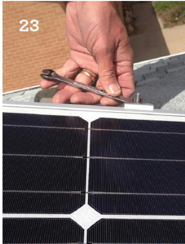
Also, in the photo, we can see that this PV installation is using monocrystalline silicon PV modules as opposed to polycrystalline silicon modules. The differences in appearance and performance and the various pros and cons of these two types of modules are discussed and illustrated in [Chapter 1](#).
