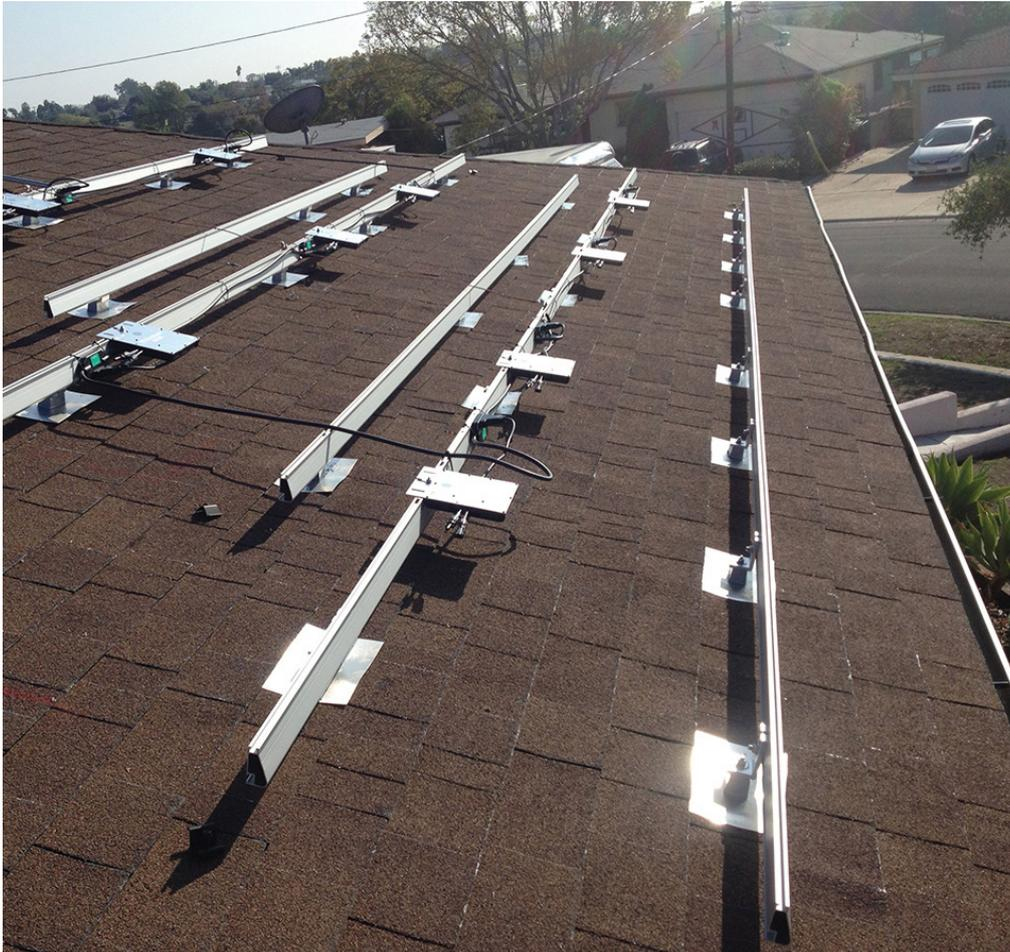
*A top view of three rows of support rails mounted on the roof with micro-inverters already attached and waiting to be connected to the PV modules.*
