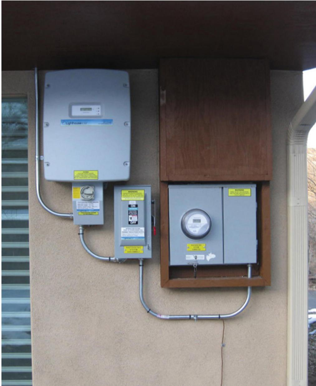
*A DC disconnect switch, a meter, and an AC disconnect switch.*
