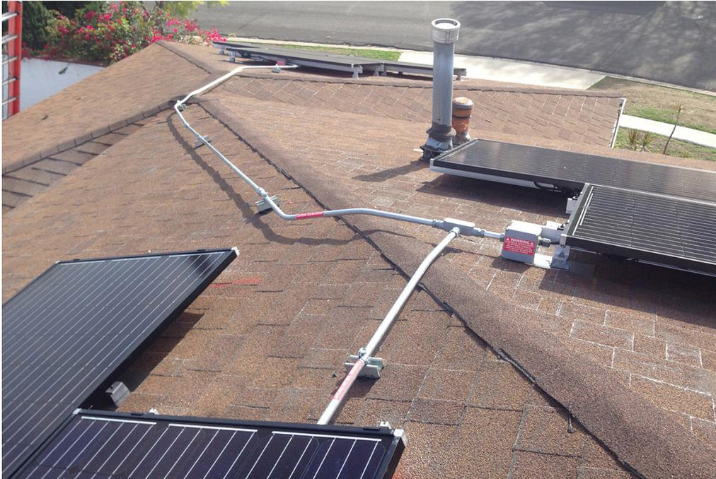
*The conduit wiring from the micro-inverters across the roof and down to the electrical control equipment.*
