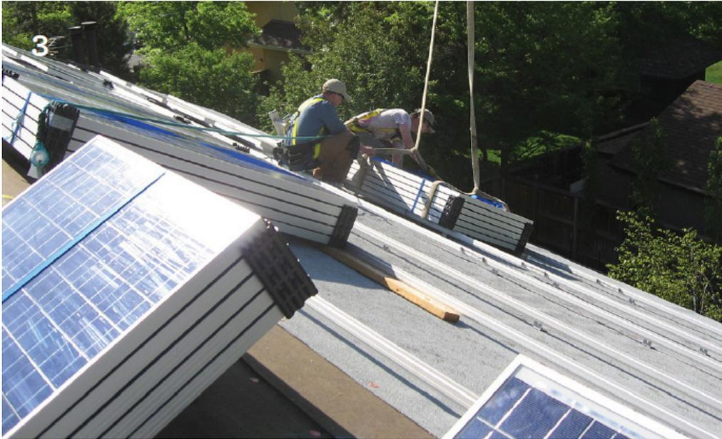
This is a fairly large installation but for smaller systems, the installer and his crew will often manually raise the PV modules up to the roof one by one using a ladder.
