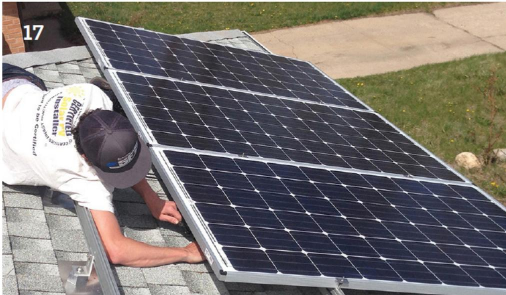
18. As shown here, it can be a bit of a tight fit to make the final connection between the leads of adjacent PV modules but the mounting support frames are engineered to allow a normal size person or worker to reach under the modules and complete the task of wiring the system.
