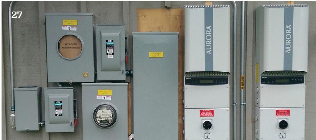
28. The photo shows the setup of the equipment area of a third, relatively simple PV solar system. Most of the same equipment items in the previous two systems are repeated here with only a few exceptions, but in this installation the current will flow from right to left.
