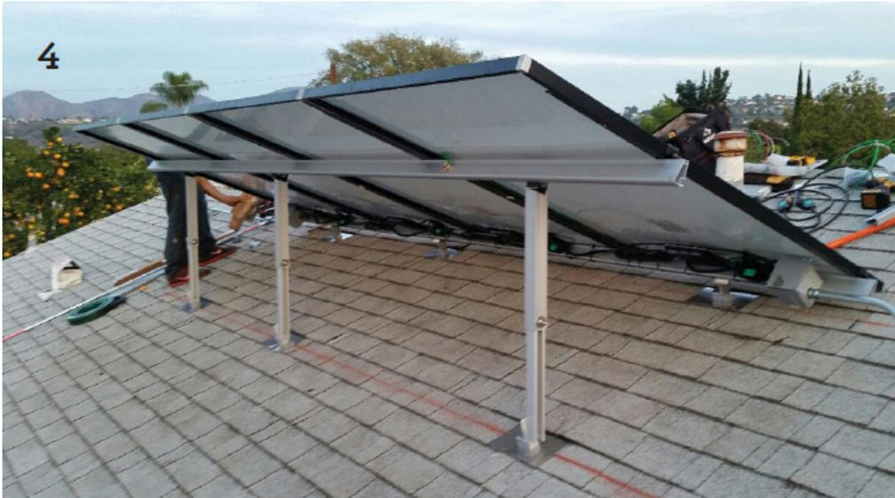
The small array above of 4 modules may be additional to modules installed on the other side of the roof to increase total system production, or, on the other hand, the main array might be mounted on this side to avoid a shading problem on the other side.
