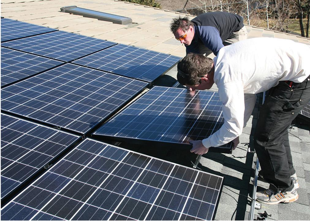
*A typical installation of poly modules that I estimate will have an installed capacity of 900 kWh/month, depending on the location of where it is installed.*
