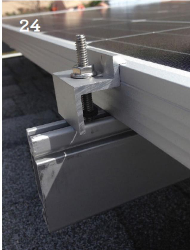
24. In the photo, we can see that the DIYer has installed one of 2 mid-clamps, getting ready to install the next panel parallel to the panel already installed.
