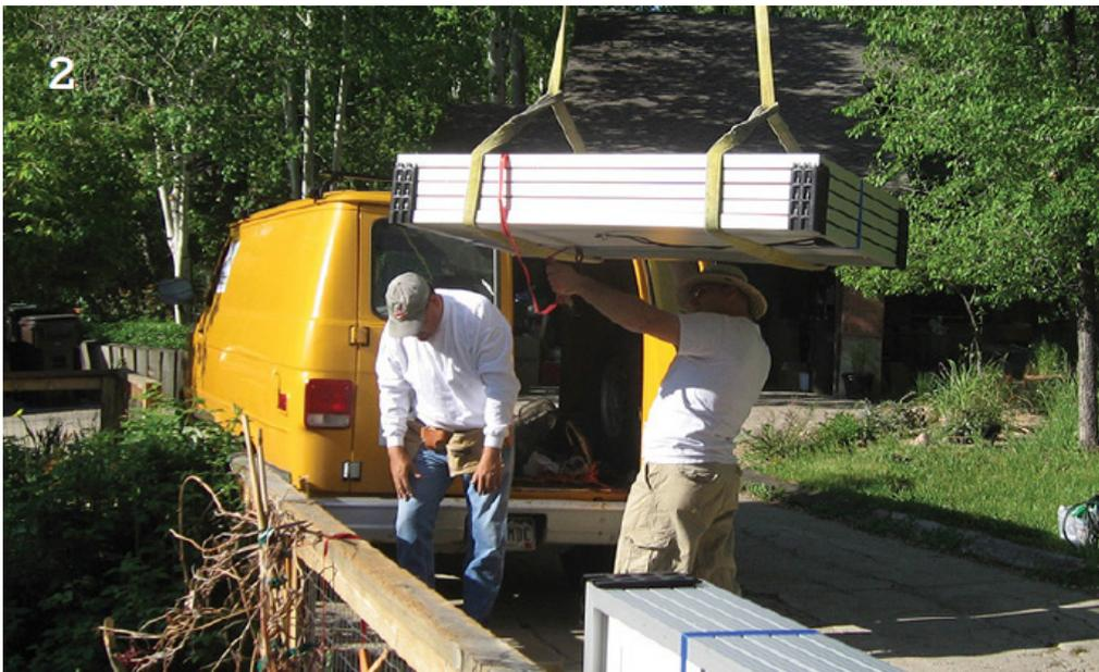
3. In the photo, we see the DIY installer and his crew guiding the crane driver and unloading the PV module packages onto the roof from the truck below. Notice that the horizontal support railings have already been installed and provide a bracing to prevent the module packages from sliding down or falling to the ground. A precautionary note: Be careful not to unload your module bundles in an
