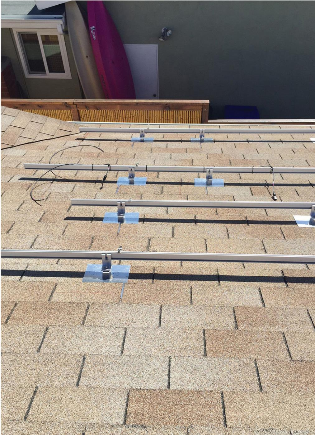
*Two rows of support rails installed and waiting for installation of the PV panels and, if applicable, the micro-inverters first go on the rails before being connected to the PV panels.*
