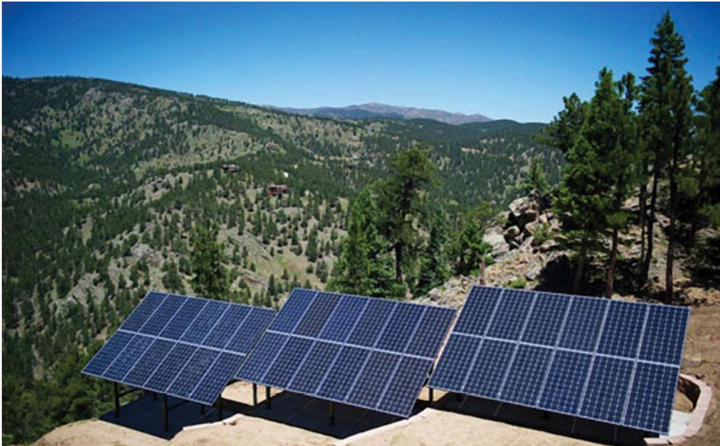
*Three arrays of 12 poly modules, each that are ground-mounted on three terraces in steep terrain. When your rooftop space is insufficient for your solar power requirements, this type of ground-mounted supplementary PV installation may be a good solution if the extra space is available somewhere behind your house.*
