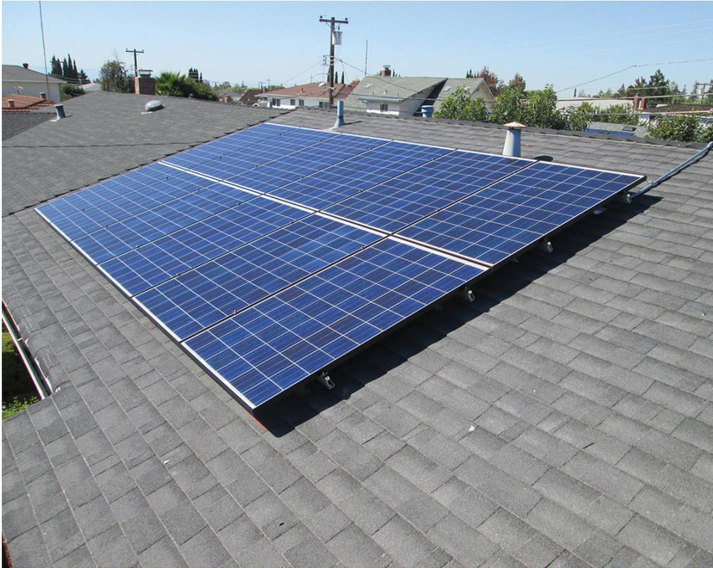
*A very typical PV solar rooftop installation of (2 rows × 6 panels) = 12 poly panels that would qualify for optimal government incentives in most states of the United States.*
