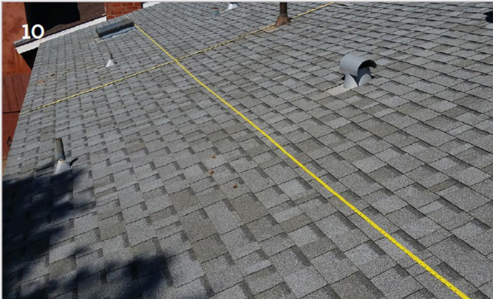
11. In the photo to the right, we see the DIY installer is taking and recording careful measurements from the edge of the roof to all the built-in roof obstructions. These measurements will enable the installer to prepare a drawing with an optimal and accurate layout for the panel array.
