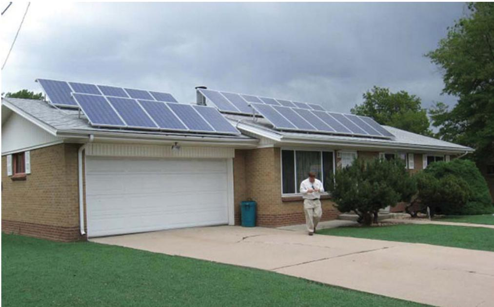
*Four arrays of five poly modules, each installed with two arrays on the main house and two equal-size arrays on the garage. We can see that the roof has a tilt of about 30 degrees and the arrays are mounted with an additional tilt of about 15 degrees for a total tilt of about 45 degrees, indicating that this house is likely located near*
