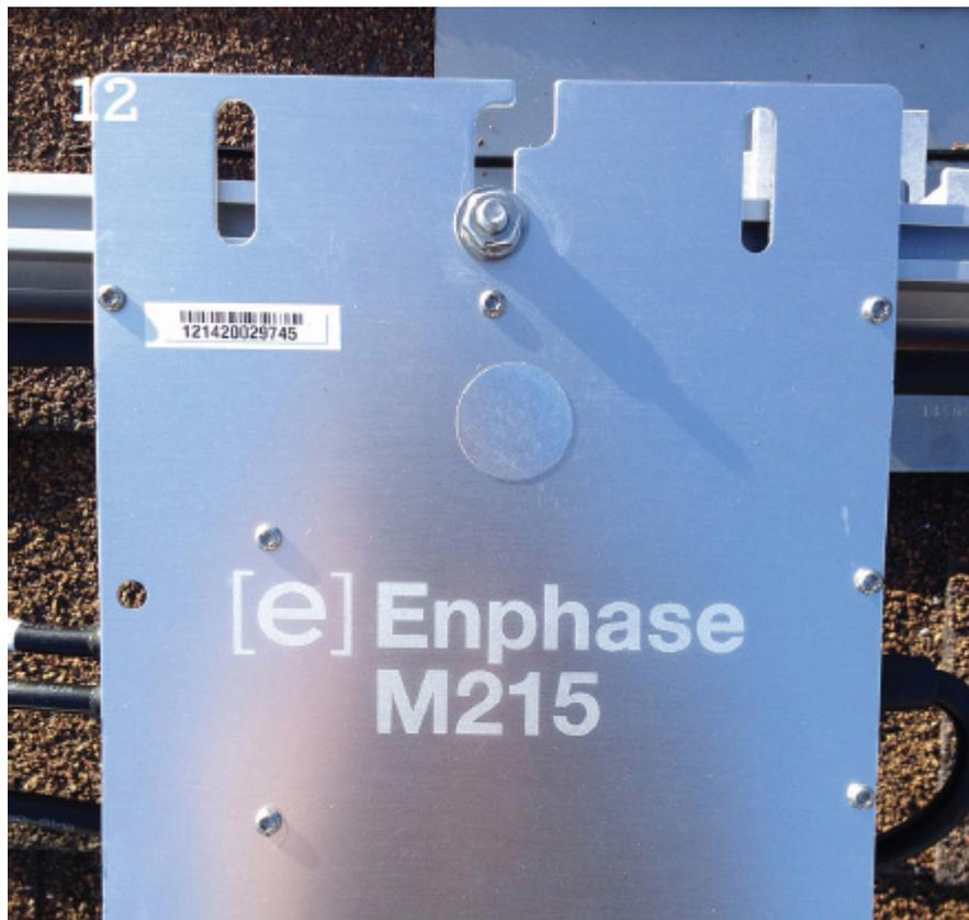
13. The photo shows a small micro-inverter with its 2 leads ready for connection. When micro-inverters are incorporated into each PV panels, you can find them
